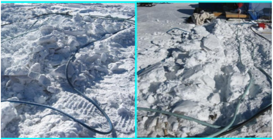
Figure 5.16 Preparing to bury cables
