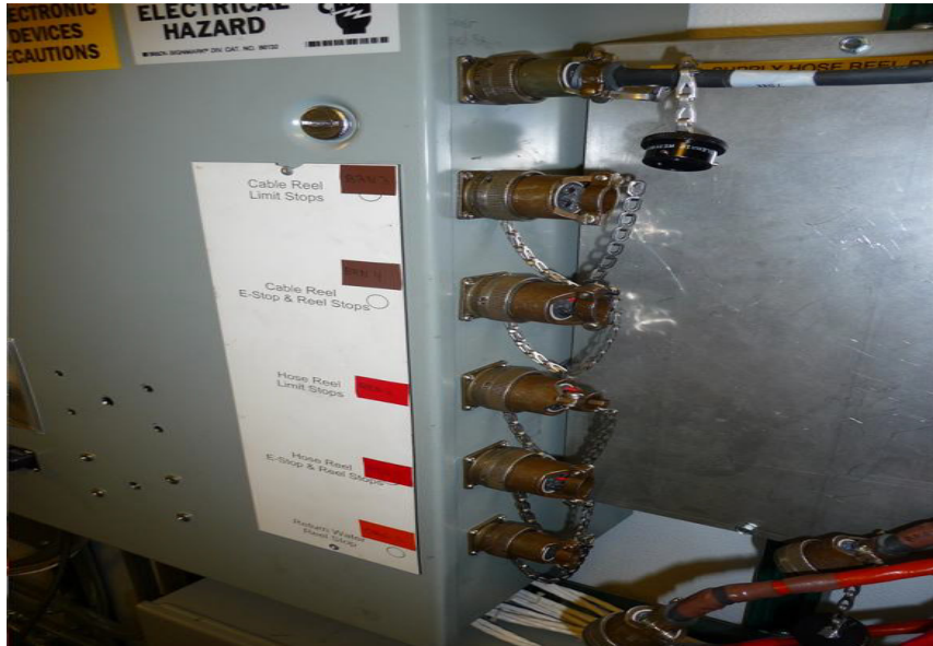
Figure 14.18 Dummy plugs installed in place of reel cables in TOS E-stop box
