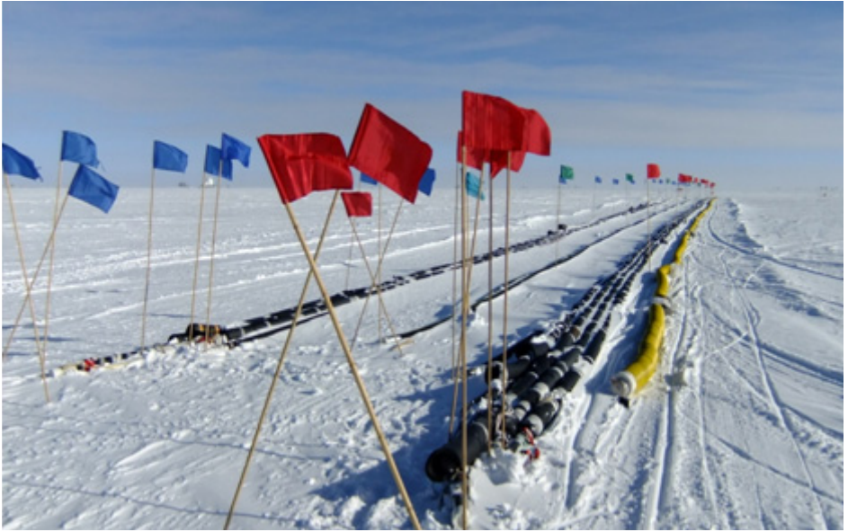
Figure 15.21 Surface hoses in their winter storage configuration
