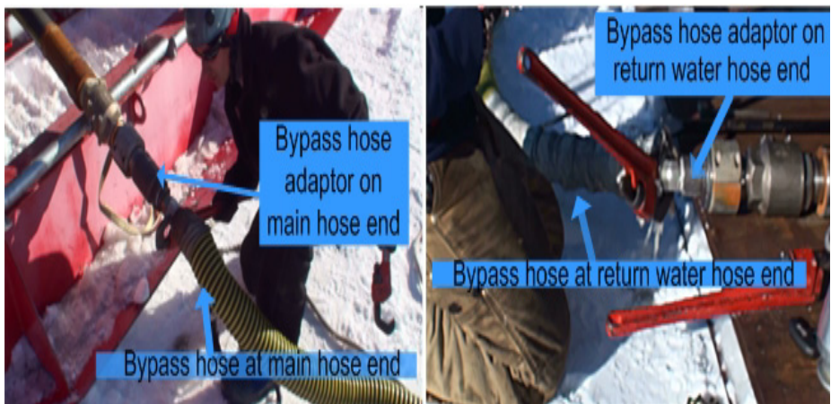
Figure 9.4 Bypass hose being disconnected from main and return water hoses
