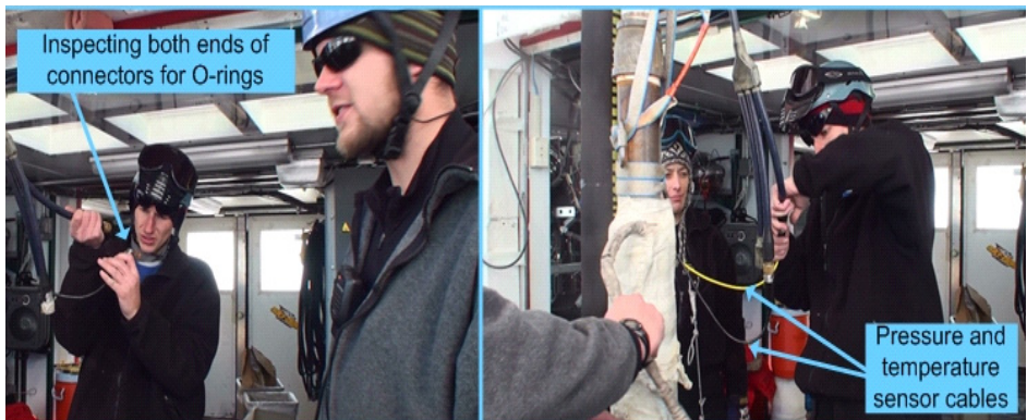
Figure 9.56 Connecting pump pressure and temperature sensors to combo cable
