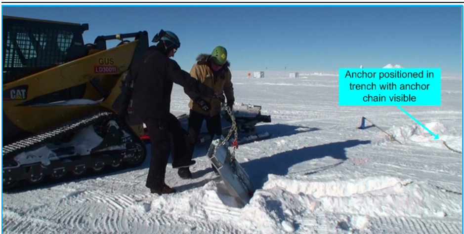
Figure 11.1 Anchors being installed in anchor trenches.
