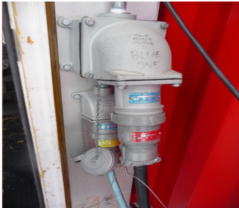
Figure 12.9 Tower hoist drum and brake cables
