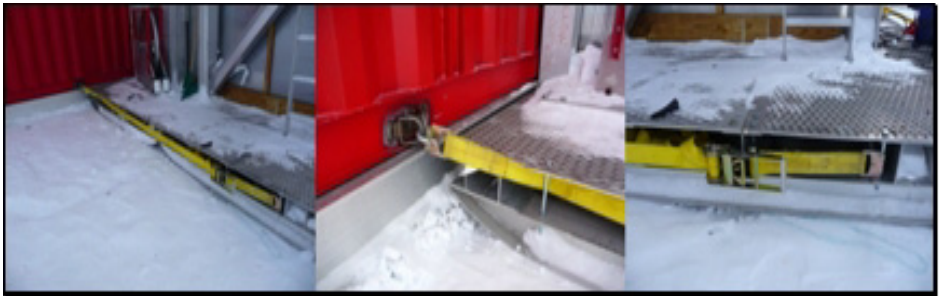
Figure 12.19 Securing of lower section of TOS to tower
