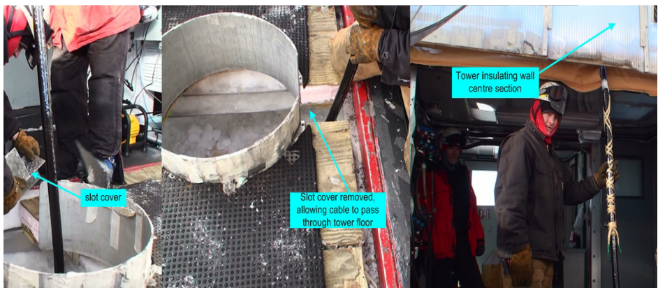
Figure 14.1 Hole slot cover being removed and tower insulating wall centre section
