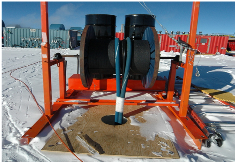
Figure 15.8 Rod Well surface hose and cable support
