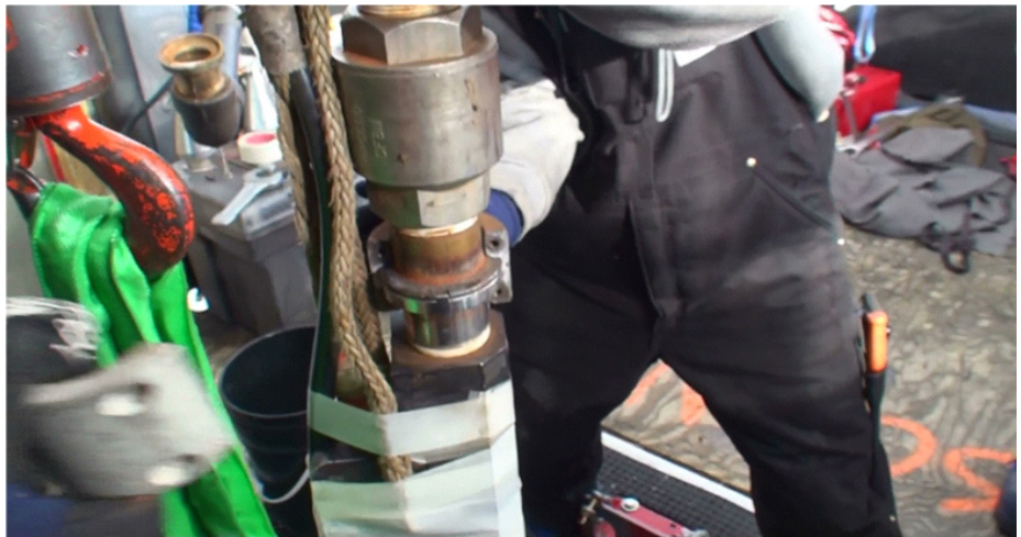
Figure 9.37 Main drill hose being connected to drill head
