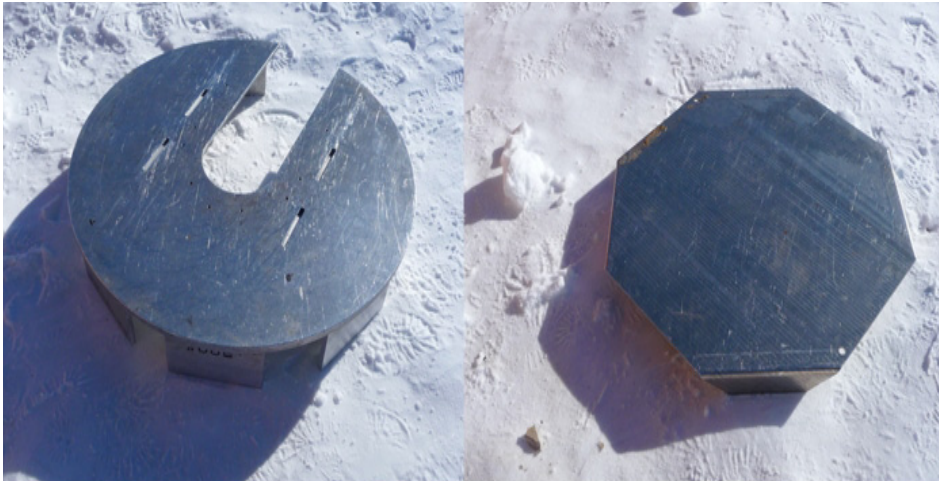
Figure 14.21 Tower hole covers
