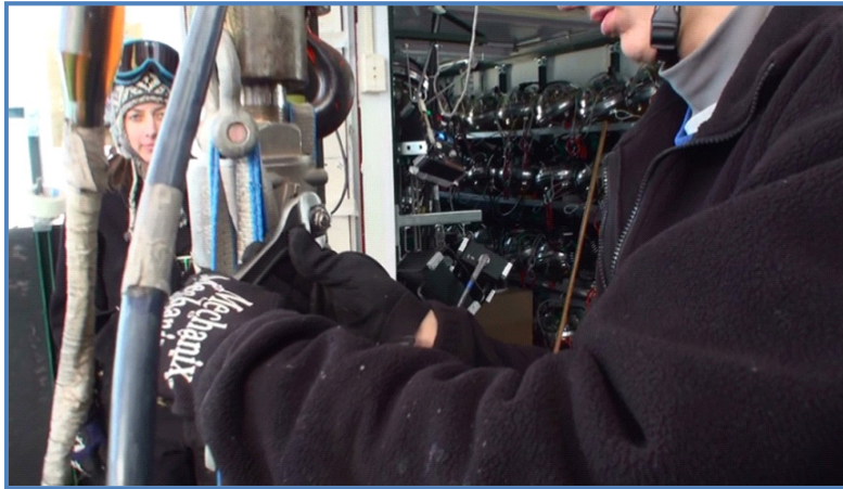
Figure 9.58 Opening return water hose outlet valve prior to lowering pump
