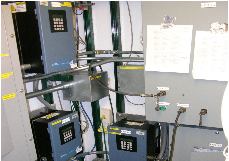
Figure 5.8 E-Stop enclosure where the E-stop cables enter and exit at the front of the cabinet
