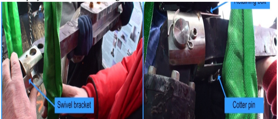
Figure 9.26 Drill head hanger being attached to drill head swivel bracket
