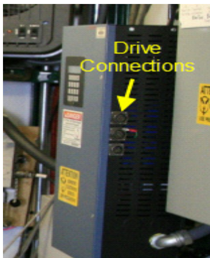
Figure 3.18 Drive showing where the drive control and I/O connectors are located
