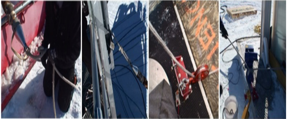
Figure 9.7 Rope setup for hauling the main hose into the tower
