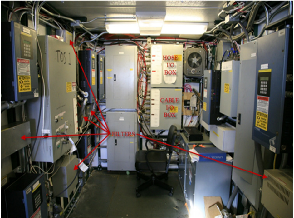
Figure 3.19 TOS drive filter locations
