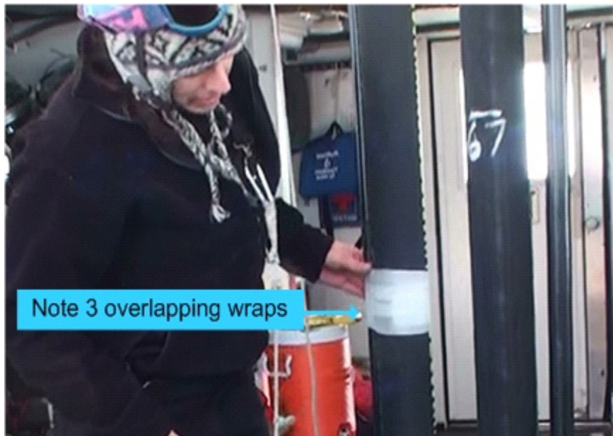
Figure 9.51 Proper taping Procedure
