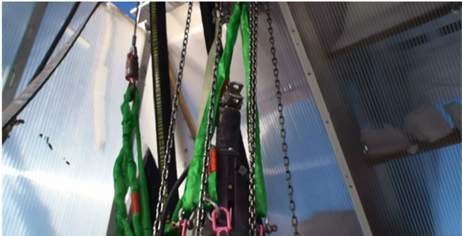
Figure 9.20 Drill head attached to chain hoist and tower hoist.
