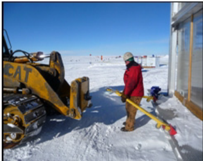
Figure 14.6 Hooking up tower tow bar to front of loader
