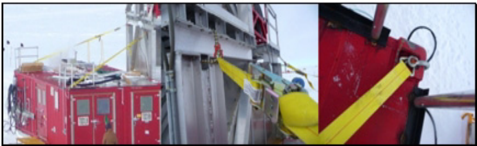
Figure 12.20 Securing upper section of TOS to tower
