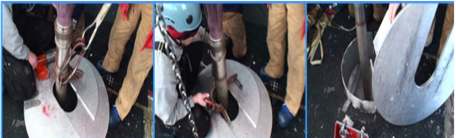
Figure 9.24 "Quick clamp", safety tether and weight stack assembly plate being removed
