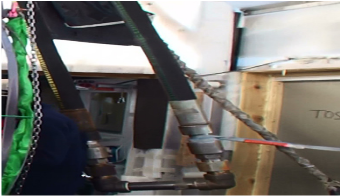
Figure 9.9 Hoses coupled together inside tower
