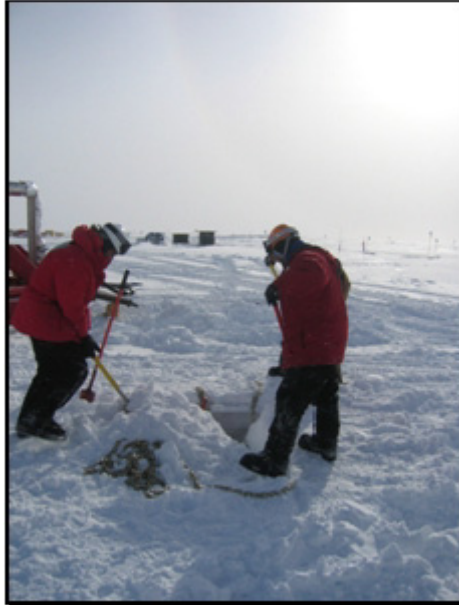
Figure 13.8 Installing reel anchors
