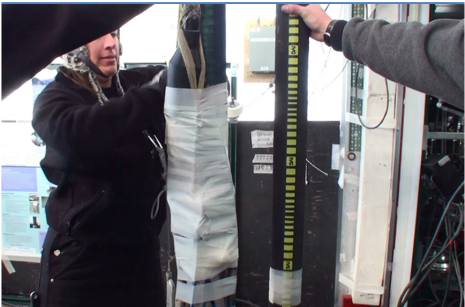
Figure 9.59 Taping submersible pump cables, connectors and slings against pump body.
