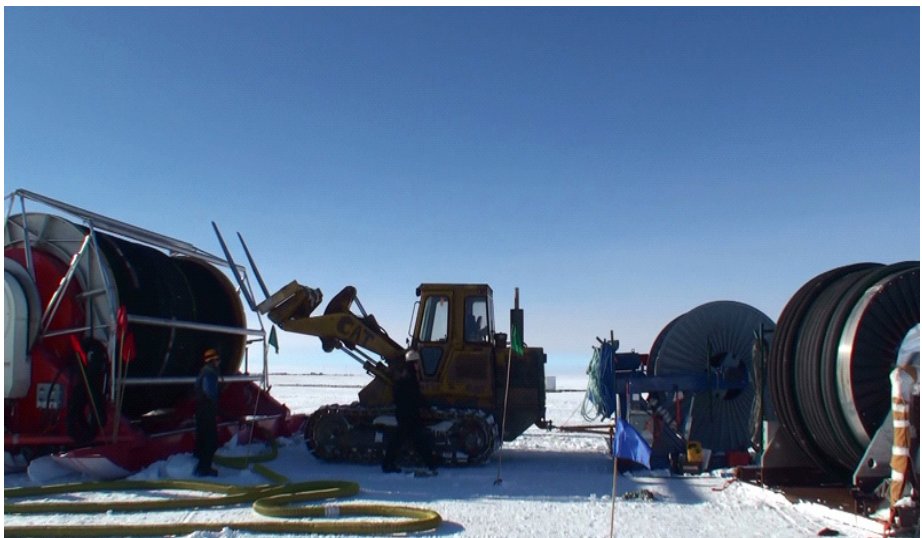
Figure 10.5 Moving deployment reel into position
