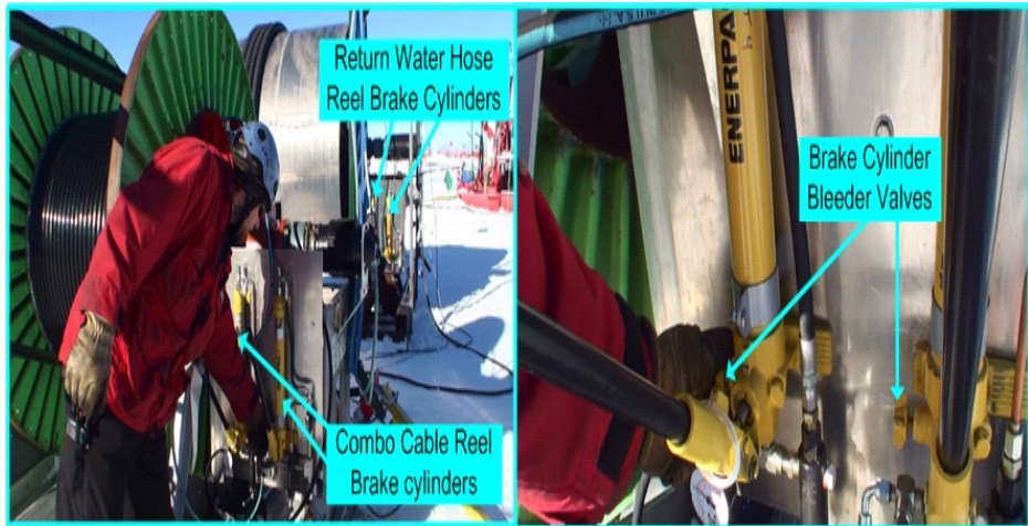
Figure 9.64 Return water pump reel and Combo cable reel brakes being applied
