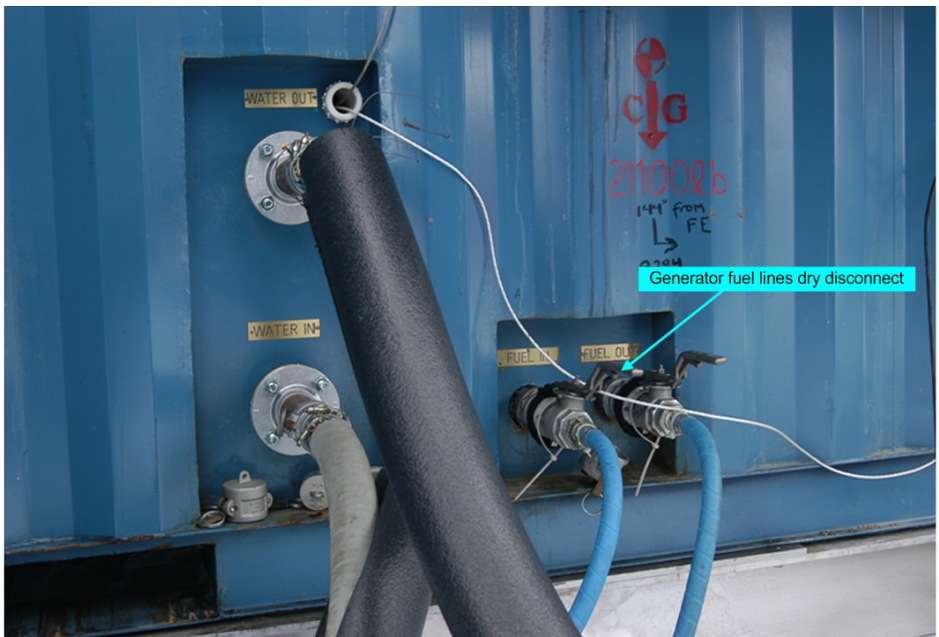
Figure 15.17 Generator fuel lines dry disconnects
