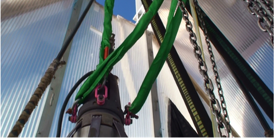
Figure 9.21 Tower hoist supporting drill head weight with chain hoist slings slack.
